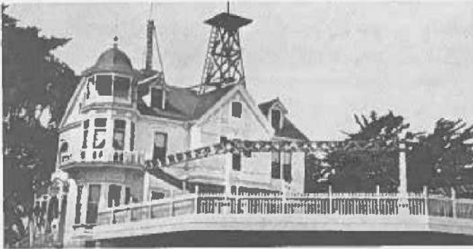
The deck that became the foundation of the Twin Inns' new dining room...
