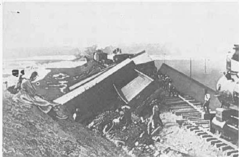
Train derailed by the flooded San Luis Rey River
