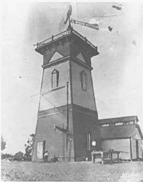
John Frazier's water tower
